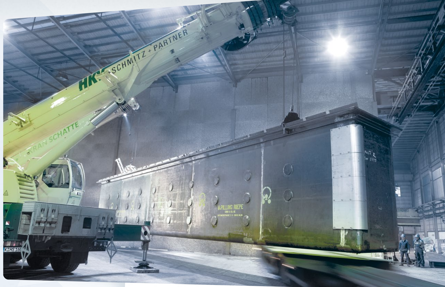
Big kettles: We galvanize components with a length of up to 19.2 metres in a single dipping operation.
